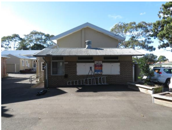
Figure 2.51 Building H, the canteen.
