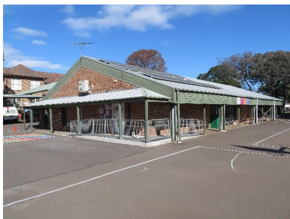
Figure 2.35 Building C, north and east elevation.
