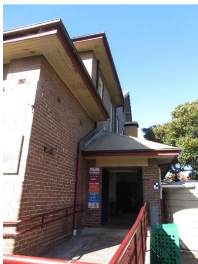
Figure 2.21 The western entrance to Building A, where the new lift and ramp would be built.
