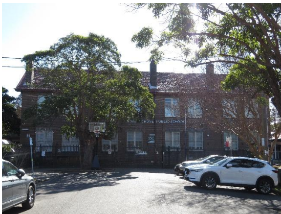
Figure 2.17 Building A, south elevation.
