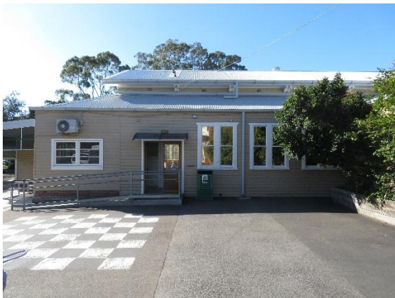
Figure 2.39 Building D, west elevation, showing the enclosed verandah.
