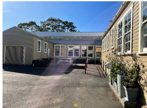
Figure 2.40 The courtyard between Building B and D, which has a timber-deck amphitheatre.
