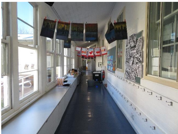
Figure 2.43 A corridor of Building D in the enclosed verandah.
