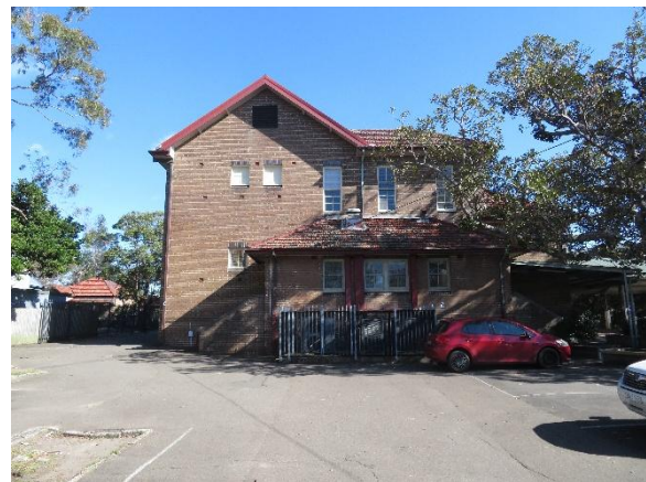
Figure 2.18 Building A, east elevation.
