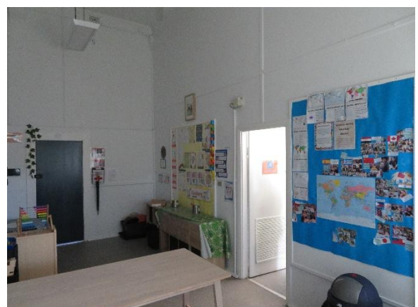
Figure 2.46 A later partition in the northernmost classroom.
