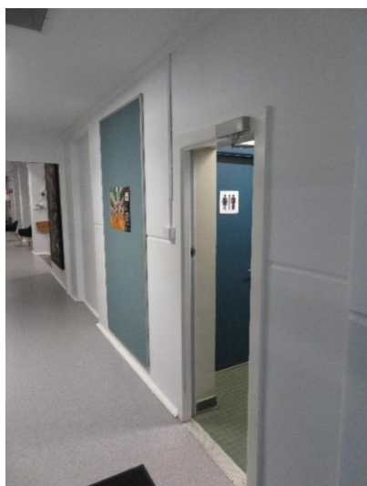
Figure 2.27 A ground-level bathroom, which would be upgraded for the project.
