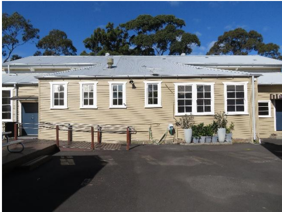
Figure 2.41 Building D, south wing.
