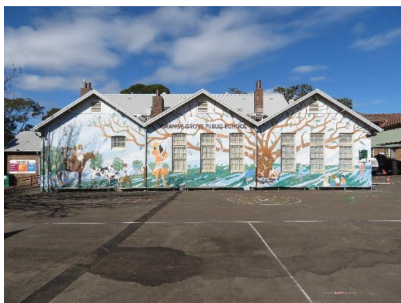
Figure 2.29 Building B, north elevation.
