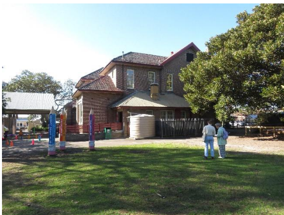
Figure 2.19 Building A, west elevation.
