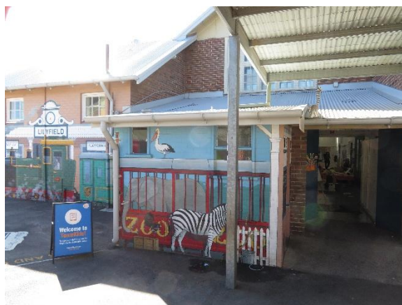
Figure 2.32 Building B, west elevation.
