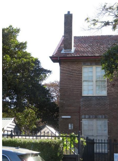
Figure 2.22 The western entrance viewed from Rayner Street.
