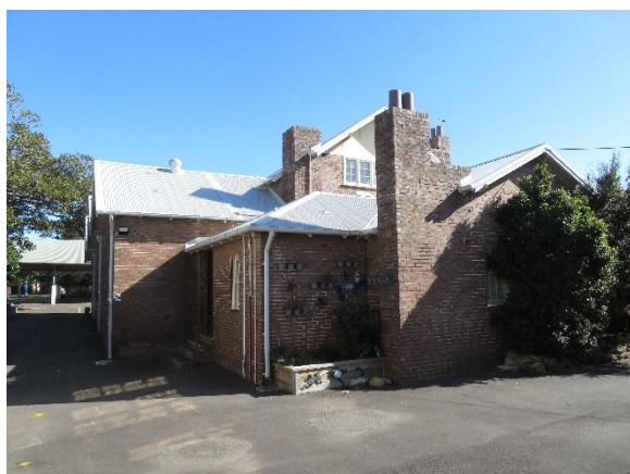
Figure 2.31 Building B, east and south elevation.
