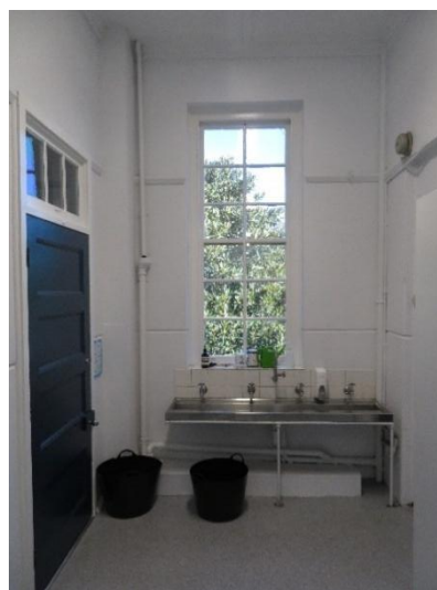
Figure 2.28 The second-level wet area, where the lift landing would be built.
