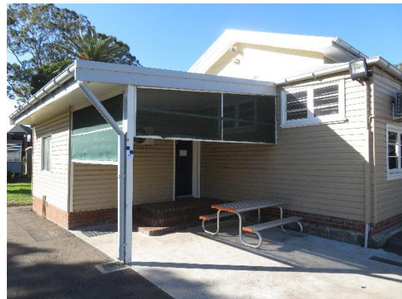
Figure 2.38 Building D, north elevation.
