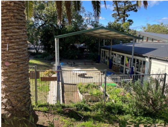
Figure 2.49 Building E, the preschool building.
