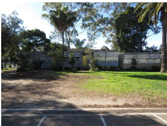
Figure 2.53 The demountable classrooms along the Balmain Road boundary.
