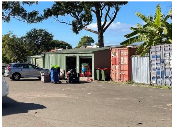
Figure 2.52 Building I, the storage shed.
