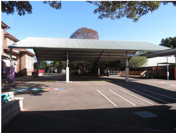
Figure 2.56 The COLA between Buildings A and C.
