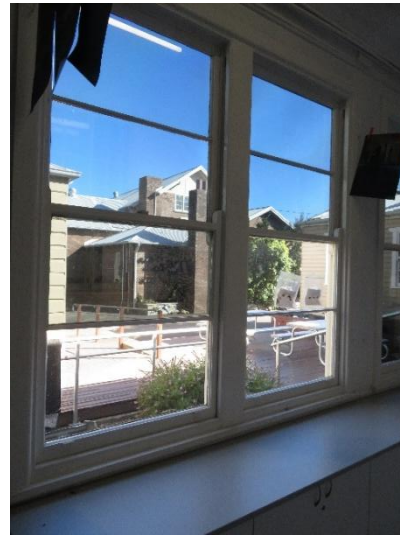
Figure 2.48 Early double-hung timber sash windows of the enclosed verandah.
