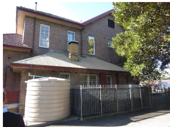
Figure 2.20 Detail of the west elevation, where the new lift would be installed.
